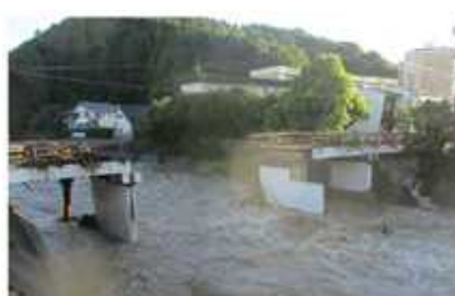
Figure 5: Futamata River (Shizuoka prefecture)
